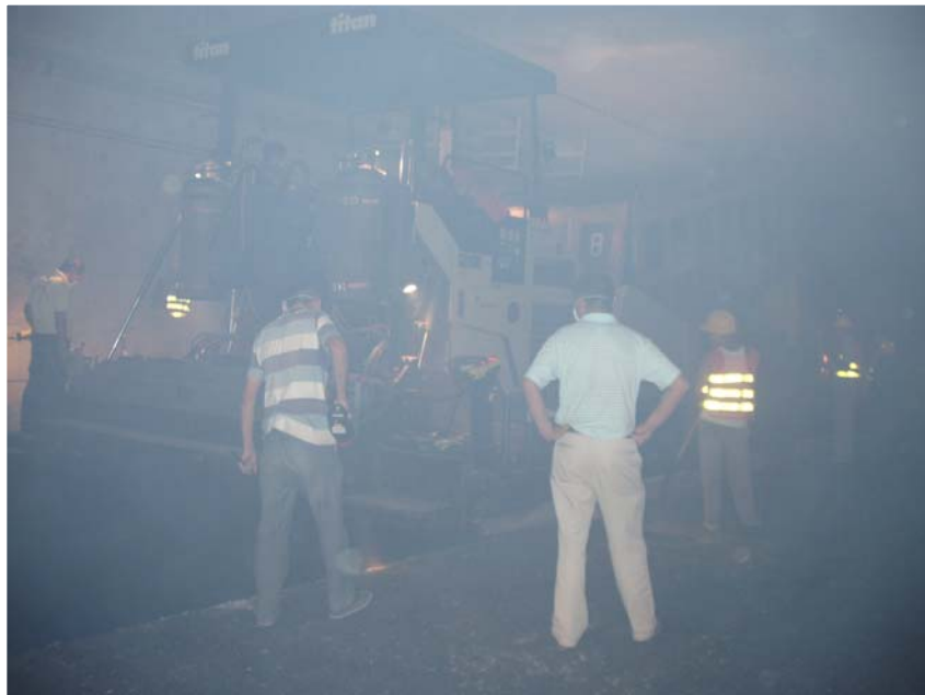
Tunnel Paving Evotherm on the left, HMA on the right
