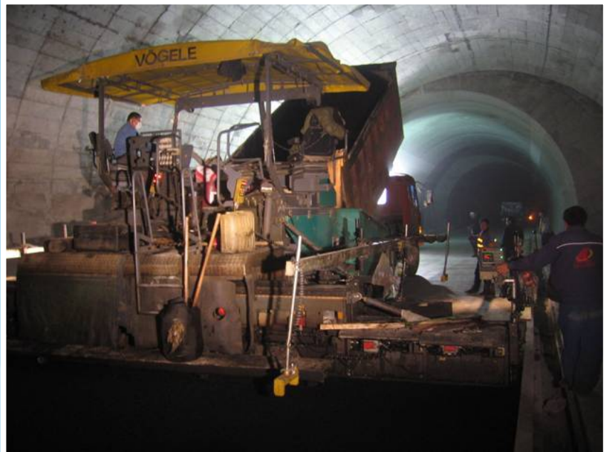
Tunnel Paving Evotherm on the left, HMA on the right
